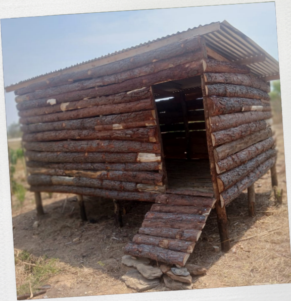
February 2026: Goat house construction
