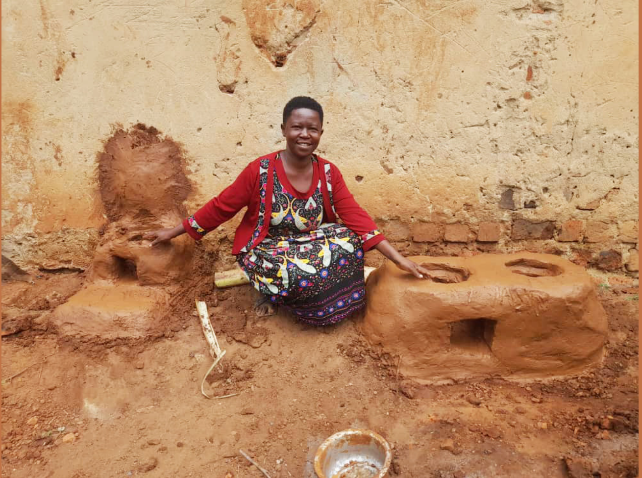
Winny with an energy efficient mud stove the group constructed during PDC training.
